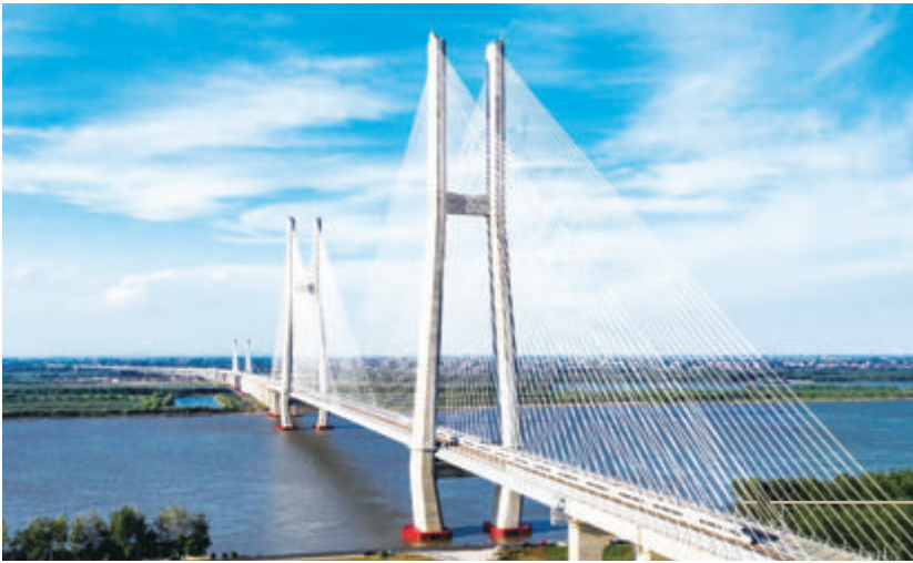
● 鳊鱼洲长江铁路大桥 Bianyuzhou Yangtze River Bridge
