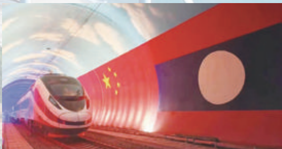
澜沧号列车穿越中国中铁建设的中老铁路友谊隧道国界段 Lancang train crossing the national boundary of the China-Laos Railway Friendship Tunnel constructed by CREC
