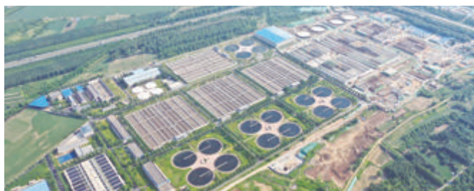
• 中国中铁建设的沈阳南部污水处理厂，为东北地区规模最大，获评全国市政金杯示范工程 Shenyang South Sewage Treatment Plant constructed by CREC, the largest sewage treatment plant in Northeast China, won the National Municipal Golden Cup Demonstration Project
