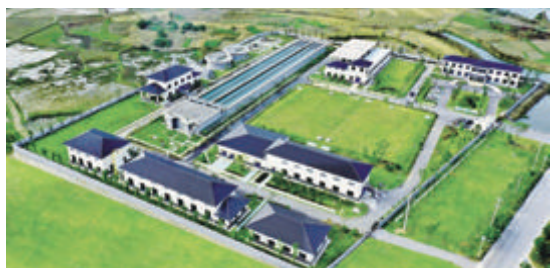
• 中国中铁建设的枞阳县农村自来水并网工程项目，总供水规模13万吨每日 Zongyang County Rural Water Supply Grid Connexion Project constructed by CREC, with a total water supply capacity of 130,000 tonnes per day
