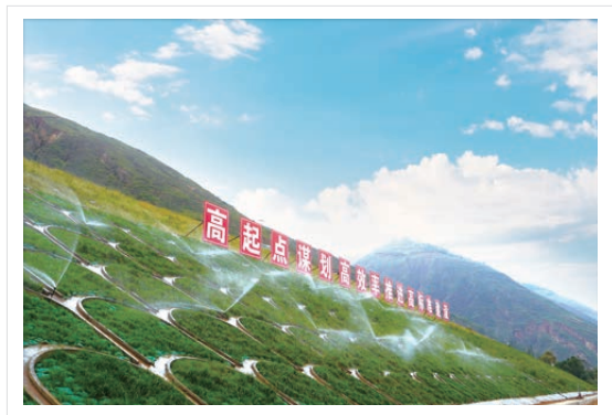
边坡绿化自动喷淋系统 An automatic spraying system for side slope greening
